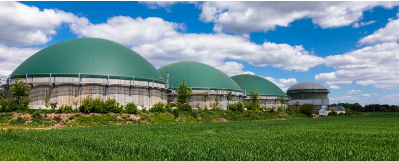
FIG. 3: ANAEROBIC DIGESTION PLANT
